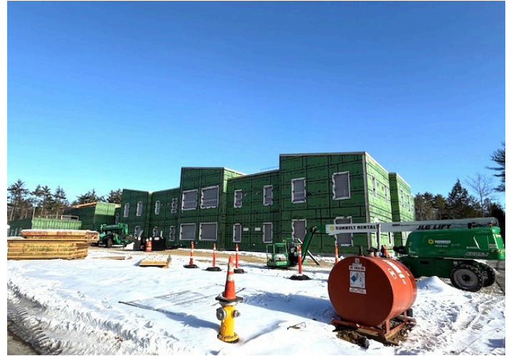
Construction of the York County Recovery Center, December 2025
